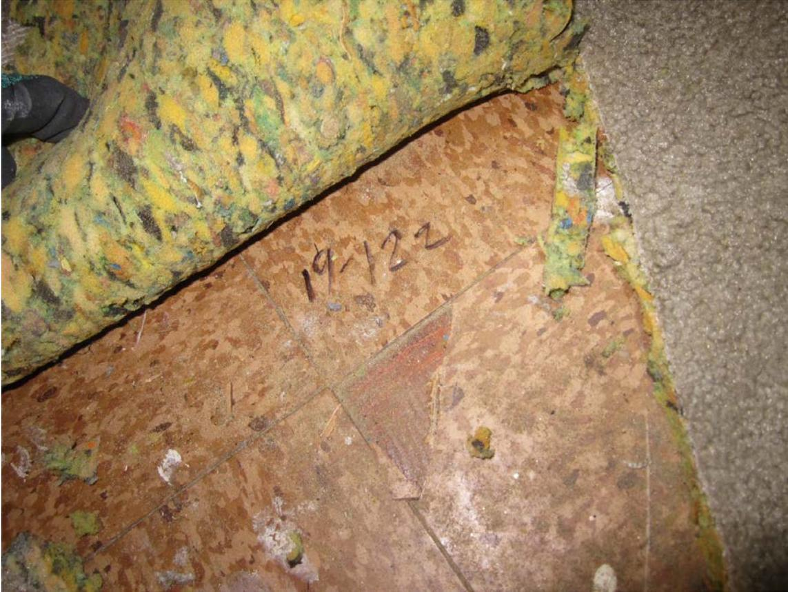
*Figure 8: 9" x 9" Floor Tile and Mastic (Greenbrook)*
