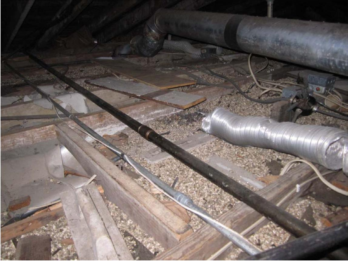
*Figure 9: Vermiculite and HVAC Paper (Greenbrook)*
