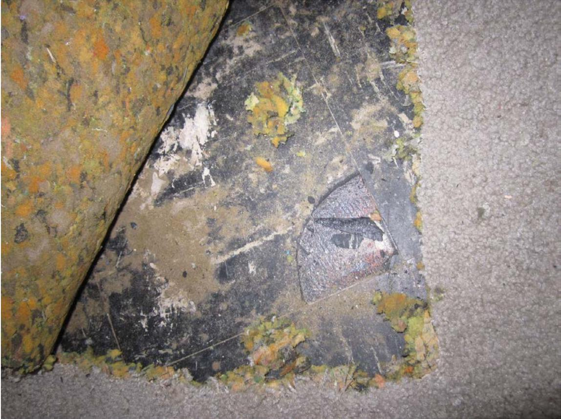
*Figure 4: 9" x 9" Floor tile and mastic (Greenbrook)*
