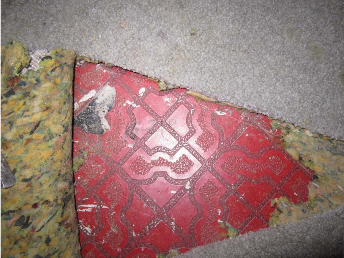
*Figure 5: 9" x 9" Floor Tile and Mastic (Greenbrook)*
