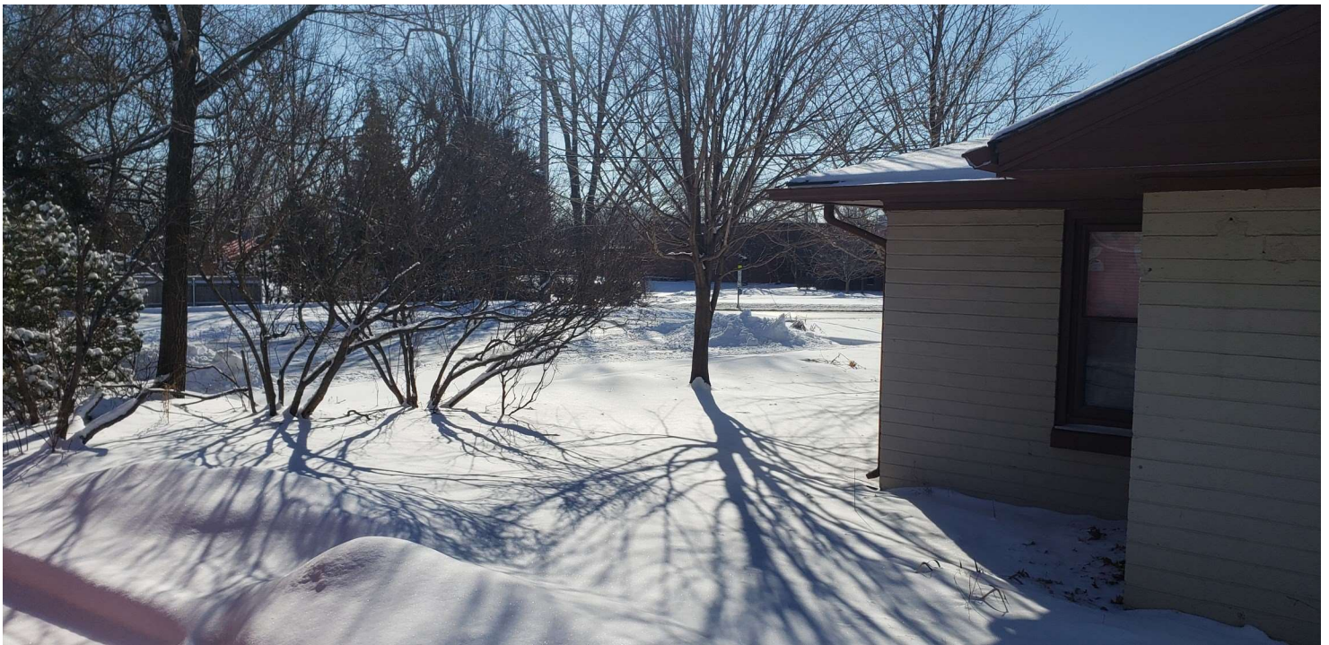
Northeast corner of building (facing southeast)
