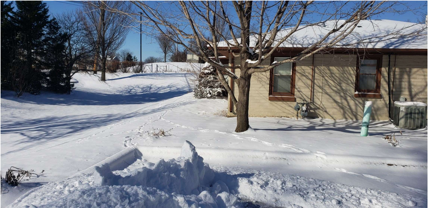
Southeast corner of building (facing west)
