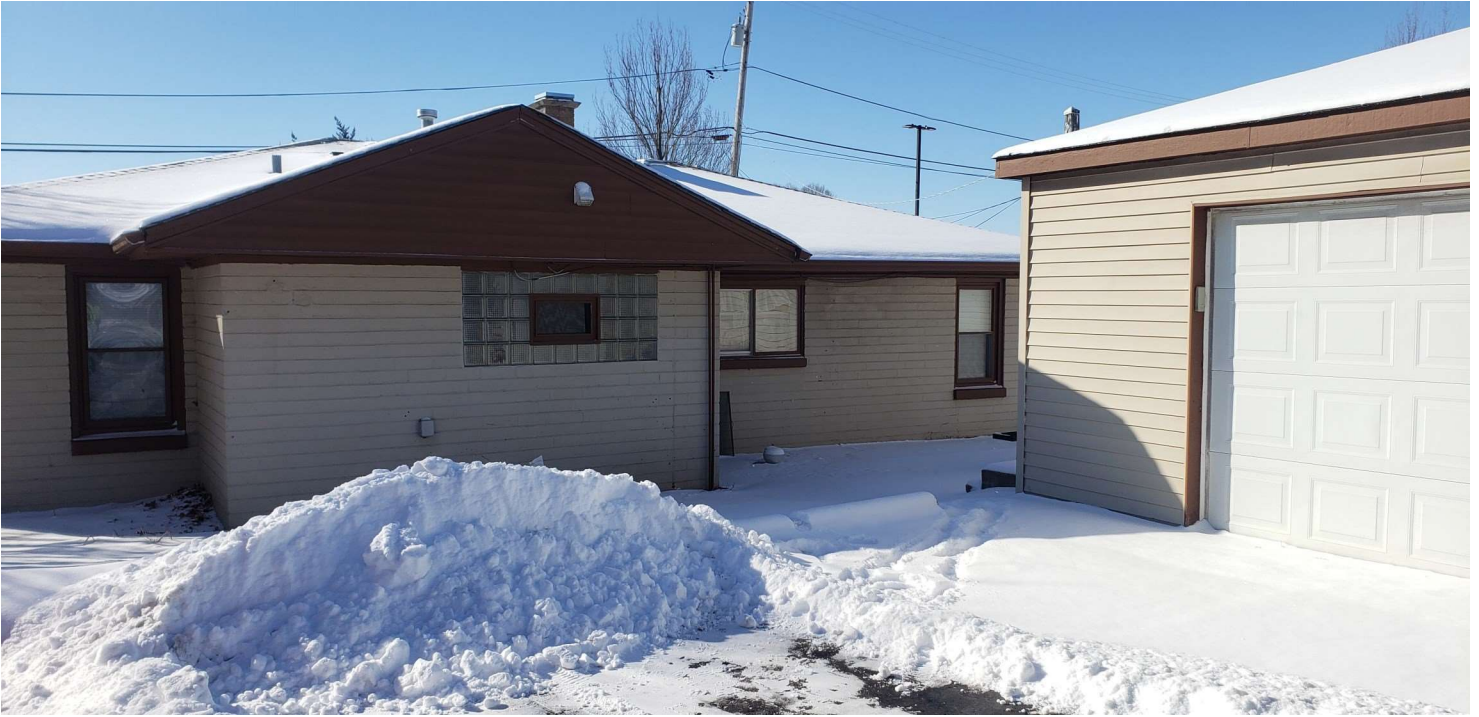
North side of building and adjacent garage (facing south)
