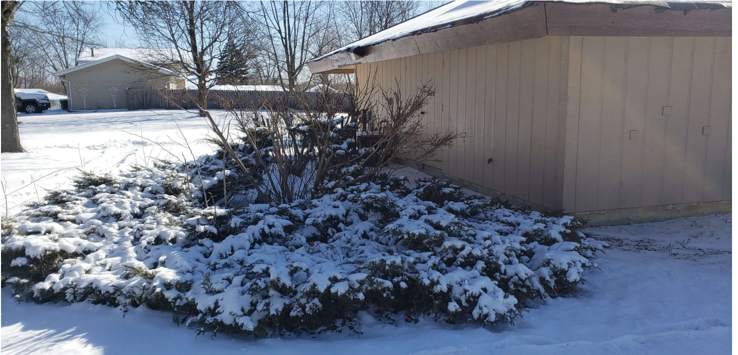
North side of building (facing east)
