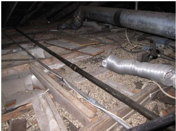
Figure 9: Vermiculite and HVAC Paper (Greenbrook)
