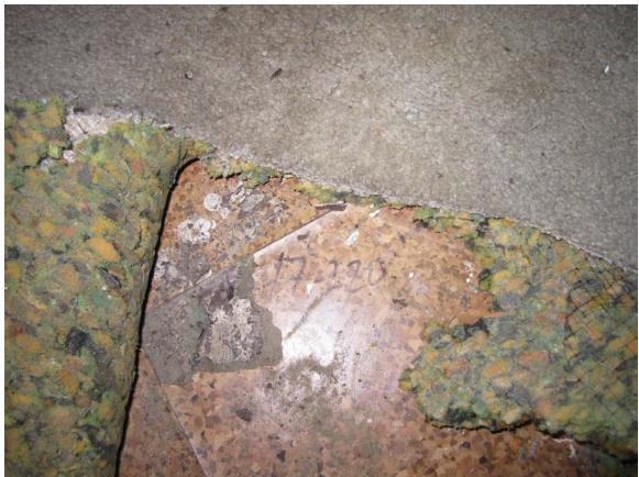
Figure 6: 9" x 9" Floor Tile and Mastic (Greenbrook)
