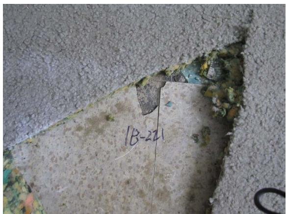
Figure 7: 9" x 9" Floor Tile and Mastic (Greenbrook)
